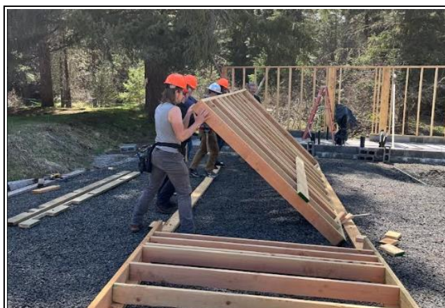
Lifting a wall is an exercise in applied physics. Many hands make work light(er)!
