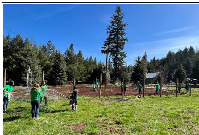
8th grade students work together to install a protective fence for newly planted fruit trees in the "Food Forest."
