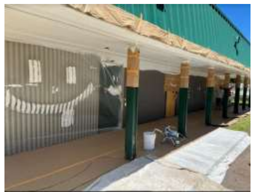
Paint finally arrives at our Elementary campus! Yay!
