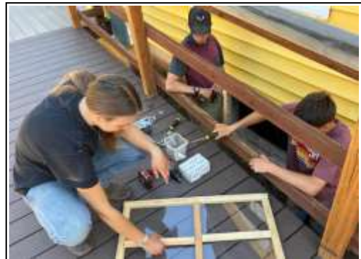
Incoming 9 th graders spend a day building and installing basement windows. 7/26/23
